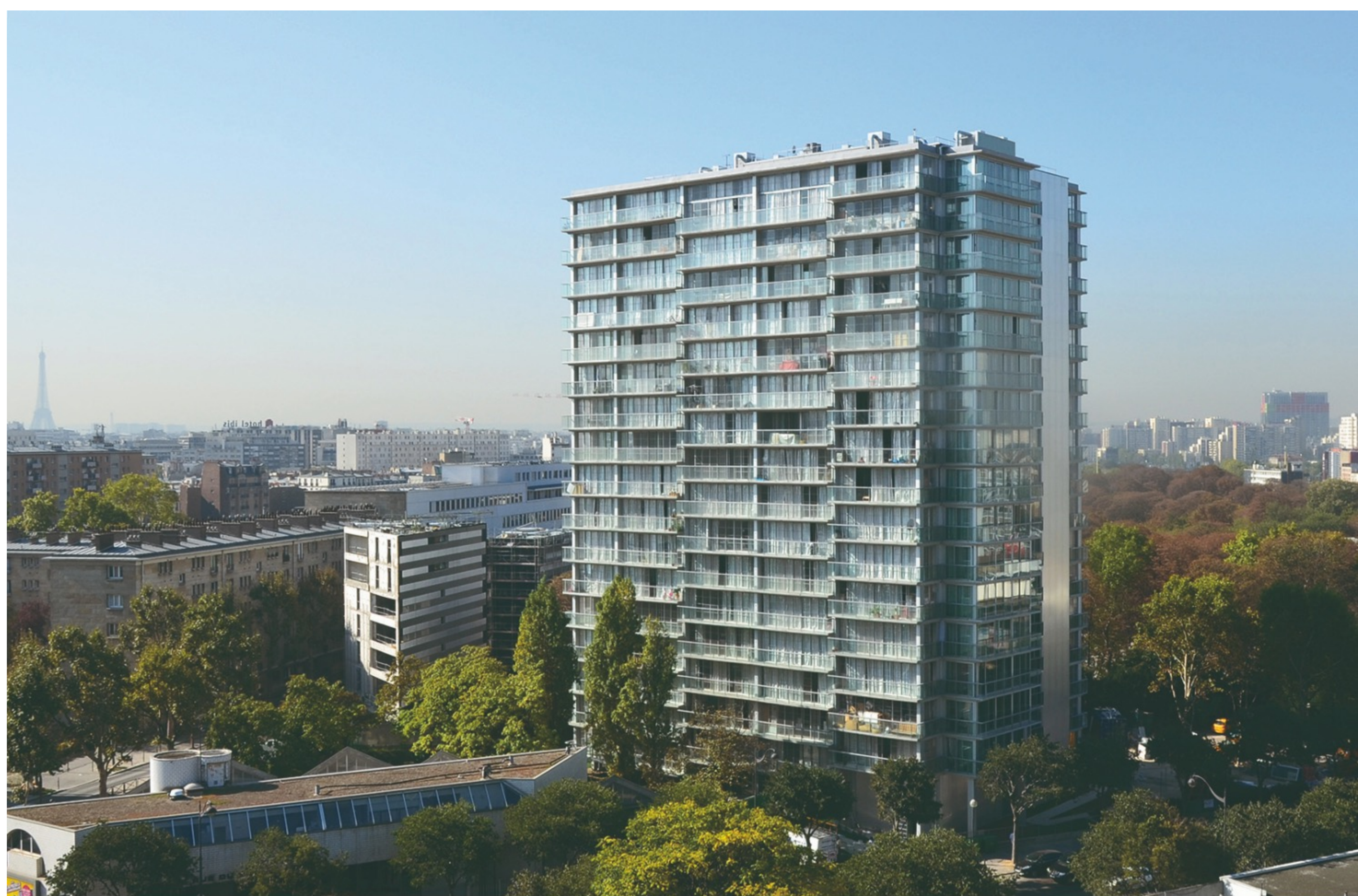
Lacaton & Vassal's careful repair and adaptation of Tour Bois le Prêtre is a successful example of using existing social housing stock Credit:Frédéric Druot
